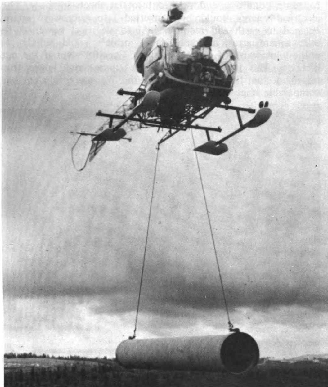
Figure 5. Small helicopters can easily position large sections of the new, light-weight, filament-wound piping in relatively inaccessible sites.
